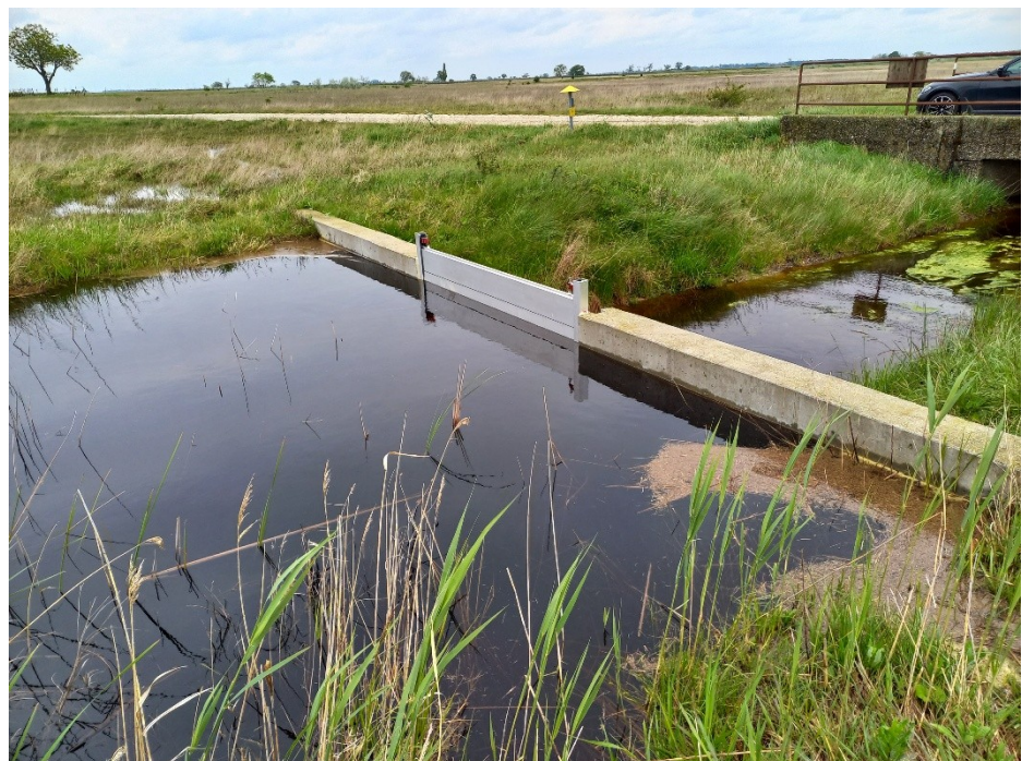
Wehranlage © Dipl.-Ing. Philipp Reiner
